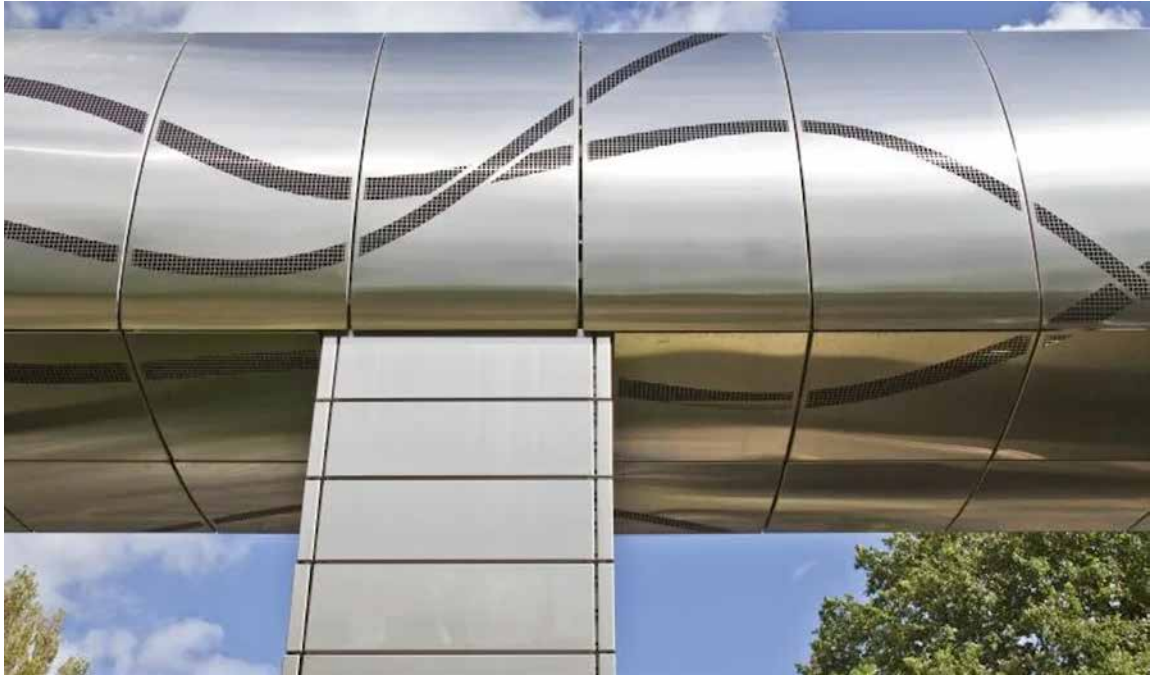
Steam Pipe Bridge, Birmingham.
