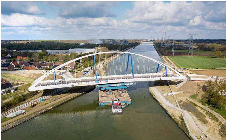
Boogbrug Albertkanaal, MeerhoutVors (B.), © DVO.
