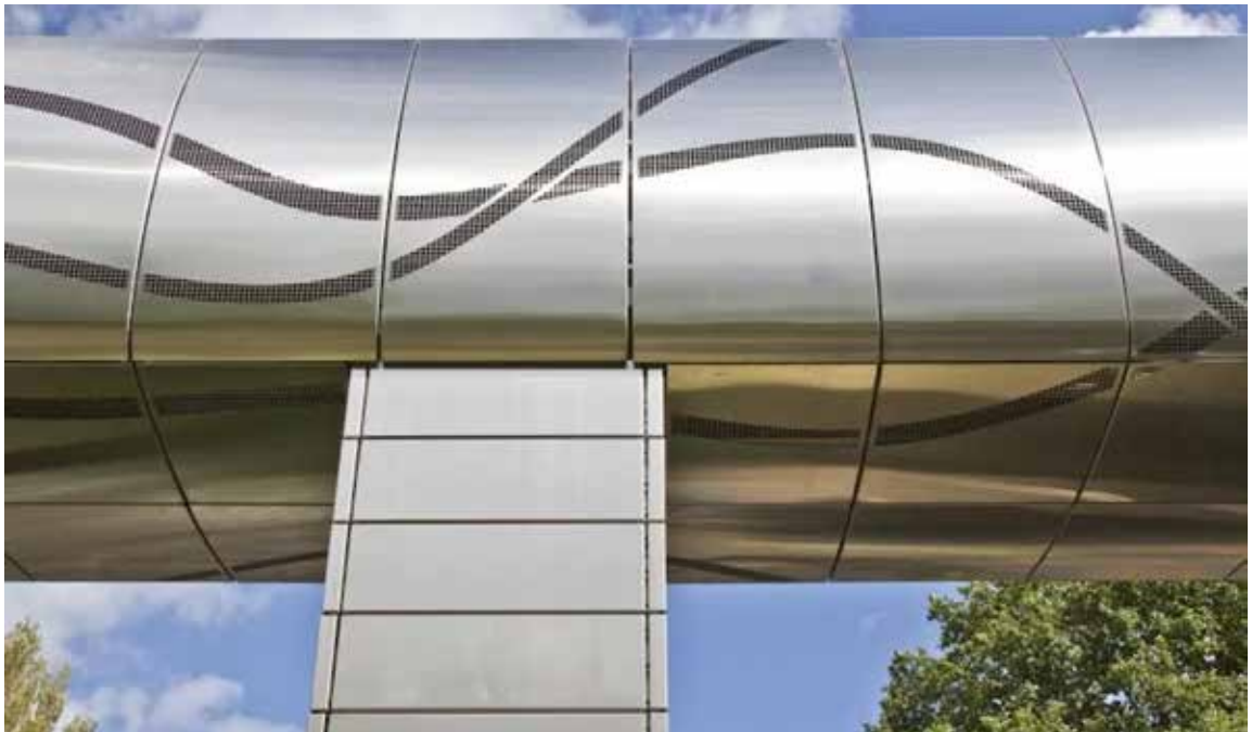
Steam Pipe Bridge, Birmingham.
