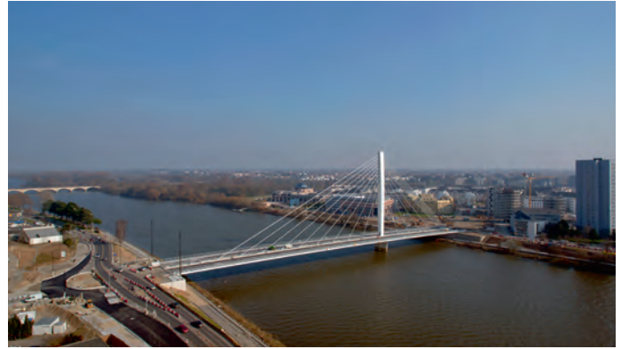
4. Brug Madeleine over de Loire in Nantes (F).
