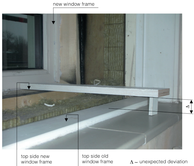
Figure 5.7: The position of the window frame in the add-on façade in relation to the existing window frame.
