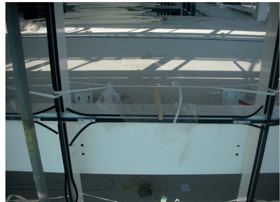
Figure 6.9: Positioning the curtain wall prior to the attachment of the interfaces.
