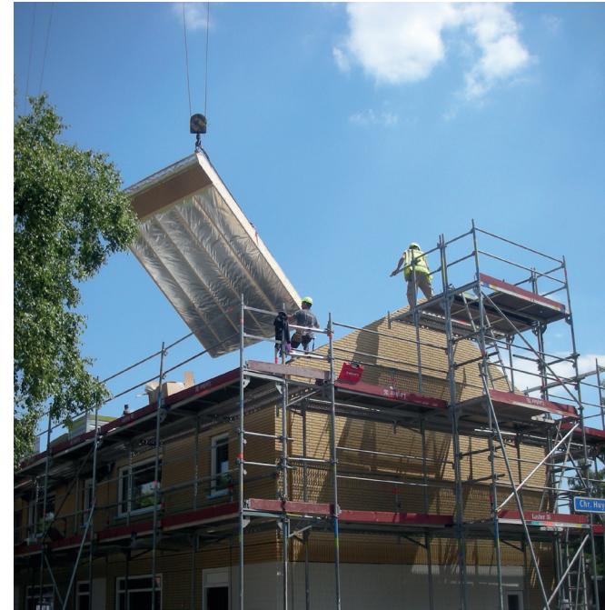
Figure 5.5: Hoisting a roof element into the desired position.
