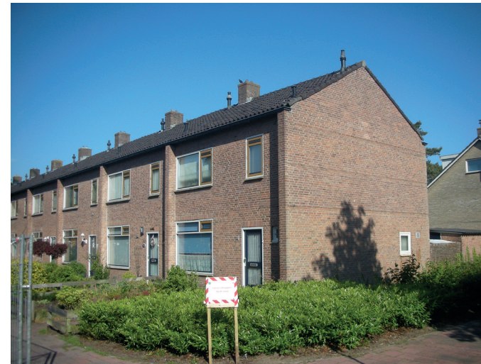
Figure 5.3: The ‘doorzon’ dwellings before transformation.
