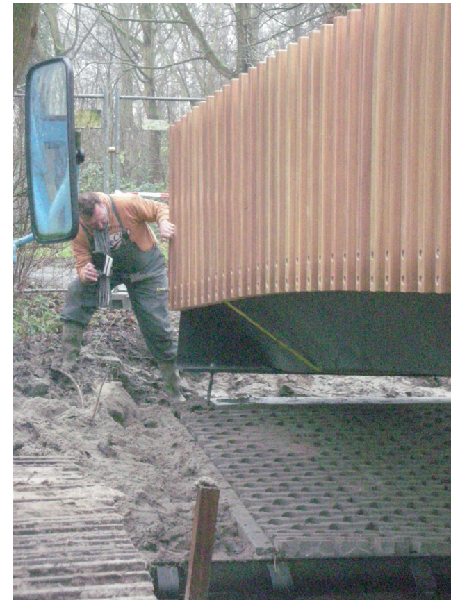
Figure 7.3: Positioning a Parks-Nature park bridge.
