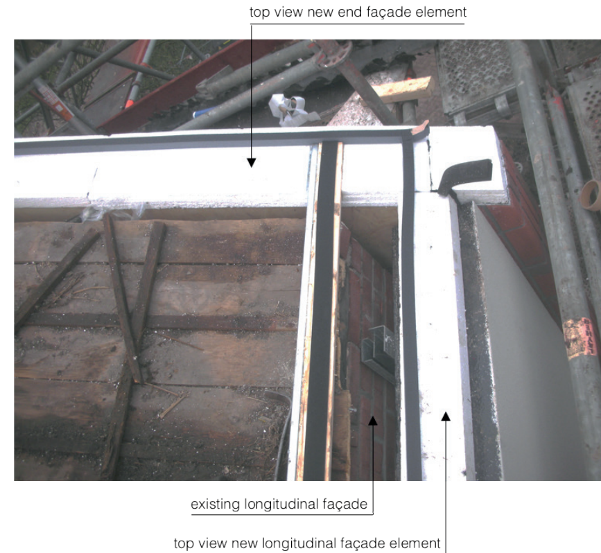
Figure 5.8: The assembly base for the sandwich panels at the location of a front façade and a side façade.
