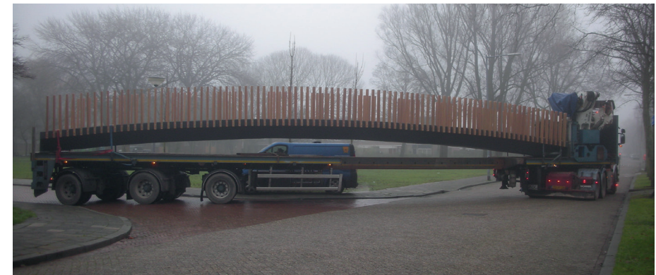
Figure 7.2: Transporting the Parks-Nature park bridge.
