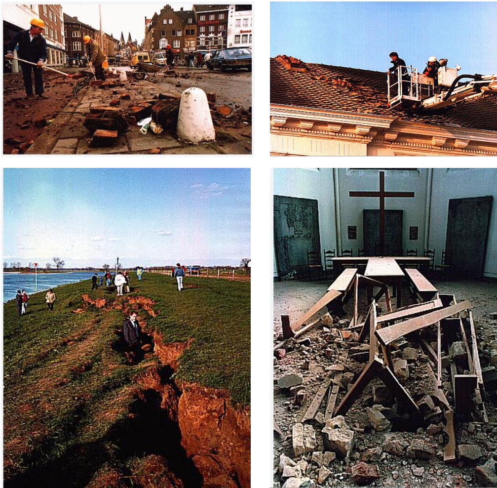
Figure 47 Observation of slight to extensive damage to buildings and failure of a canal slope as a result of the Roermond, Netherlands 1992 earthquake.
