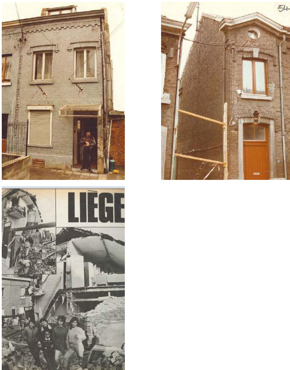
Figure 46 Observations of extensive damage and partial collapse of buildings caused by the Liege, Belgium 1983 earthquake (from EEFIT 1983).
