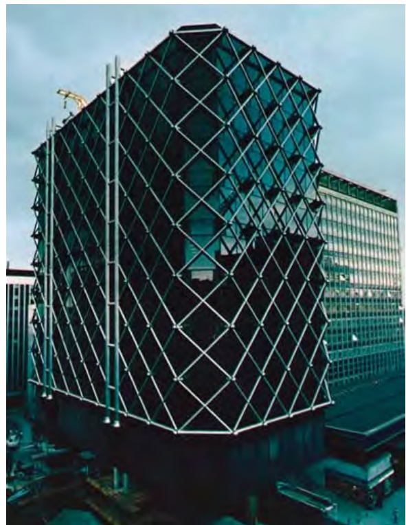
Figuur 52 Bush Lane House, London, bron [83]
